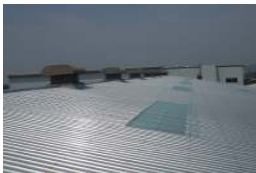
Roof with thermal insulation (Miki Plant)
