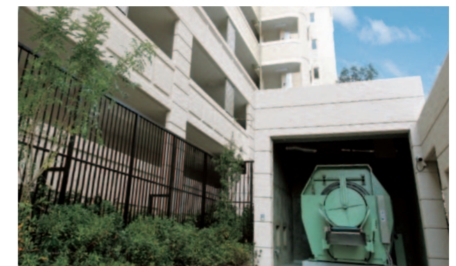
Drum-type waste storage and discharge equipment
