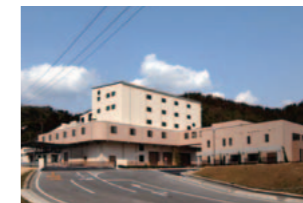
Large waste disposal facilities
