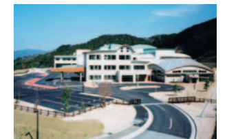
Refuse-derived fuel (RDF) processing facilities
