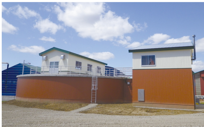
Bio gas plant
