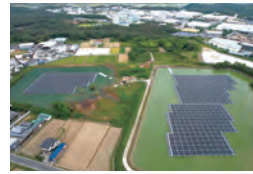
Solar Panels on a reservoir
