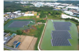
Solar Panels on a reservoir
