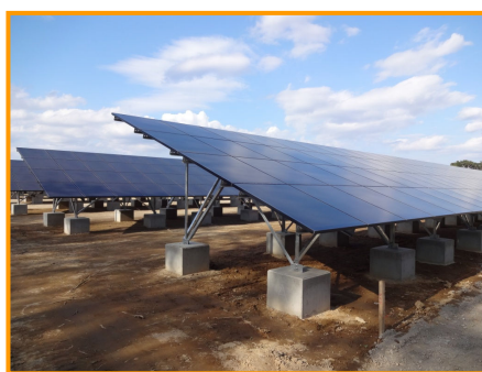
“Hachinohe Mega-Solar Power Plant” (1.5MW) (under construction)
