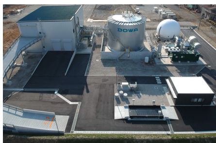
Biogas plant in Okayama
