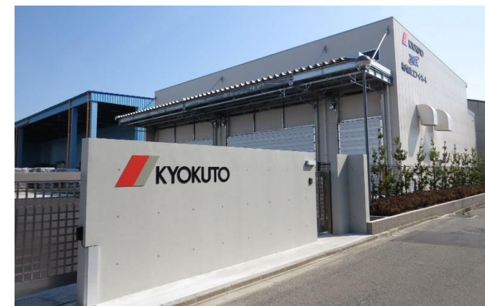
Service work building of Sendai Service Center
